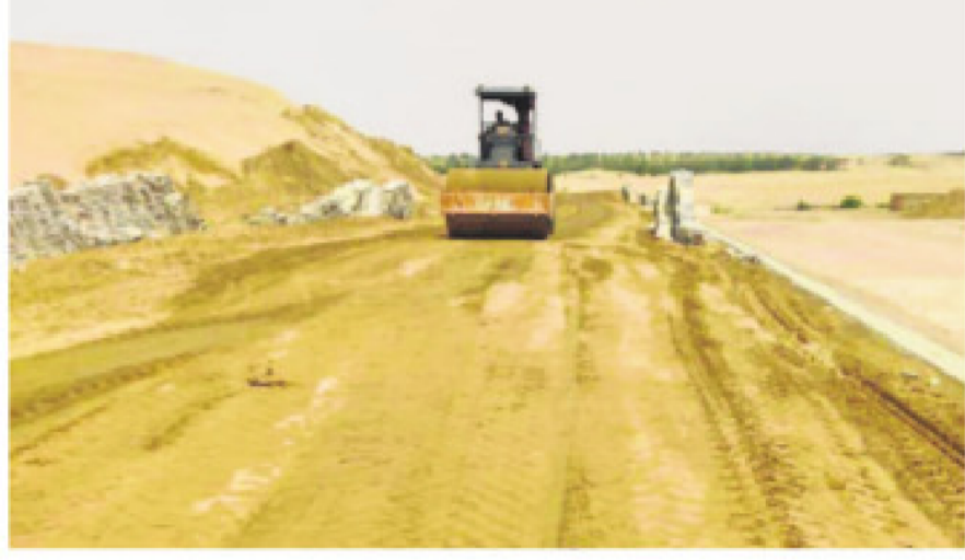
Work is underway on mega reservoir in Thar desert
